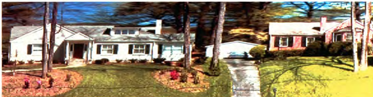
Portion of image produced from video captured while driving between five and 10 mph, using camera mounted orthogonal to path of travel with scan lines perpendicular to road surface.
